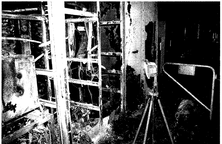
An electrical fire in a power supply at CERN will delay the restart of operations at the SPS proton synchrotron and the LEP electron-positron collider. Specialist personnel are working round the clock to repair the damage, exacerbated by acid soot contamination of adjoining areas
